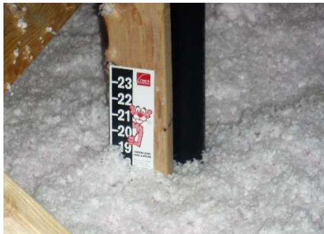
Attic insulation next to a depth measuring strip
