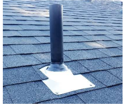
Plumbing vent flashing
