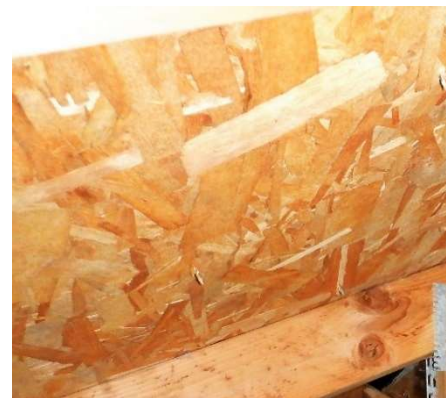
Good condition roof sheathing
