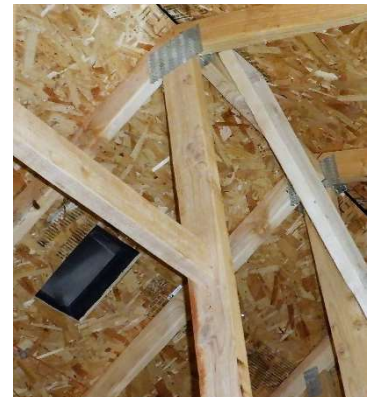
Attic roof vent
