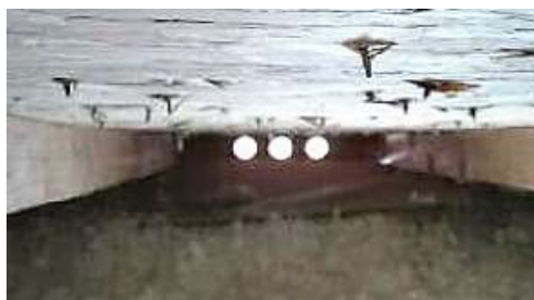
Bird block style lower attic vents
