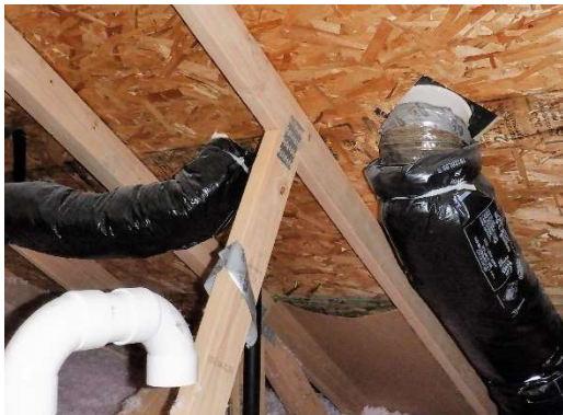
Vent penetrations through a roof
